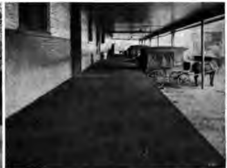
Sarco Mineral Rubber Floor, Freight Loading Dock, Libby, McNeil & Libby, Chicago
